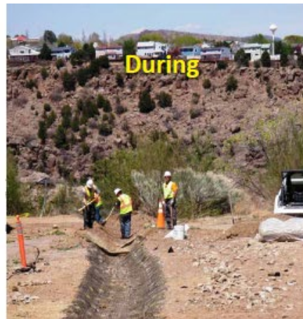
Installation of storm water controls at P-SMA-2.2
